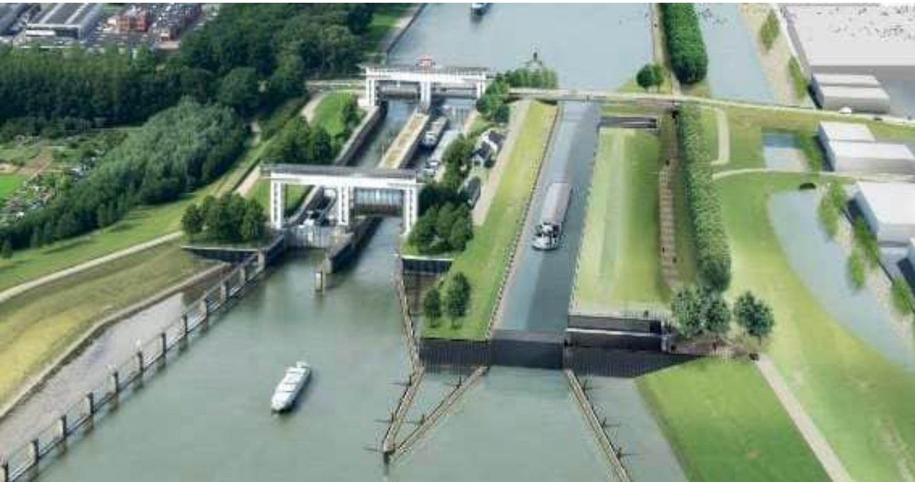
ASSET MANAGEMENT TERNEUZEN LOCK
