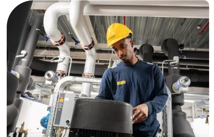
Framework contract at ASML
