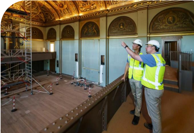
Binnenhof renovation, including Dutch Senate and Council of State
