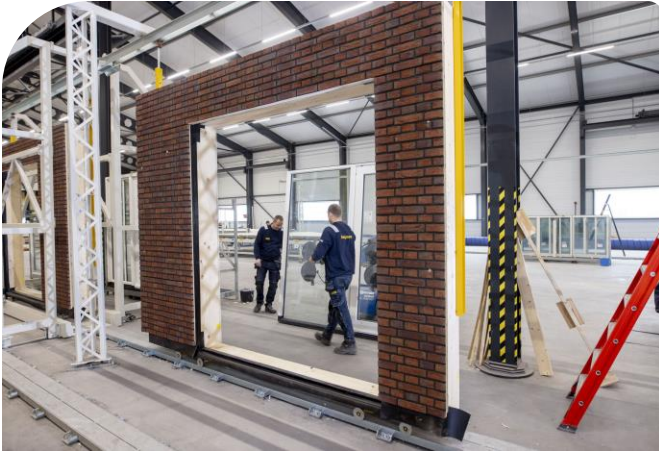
Horizon elements from the timber frame construction factory in Heerenveen
